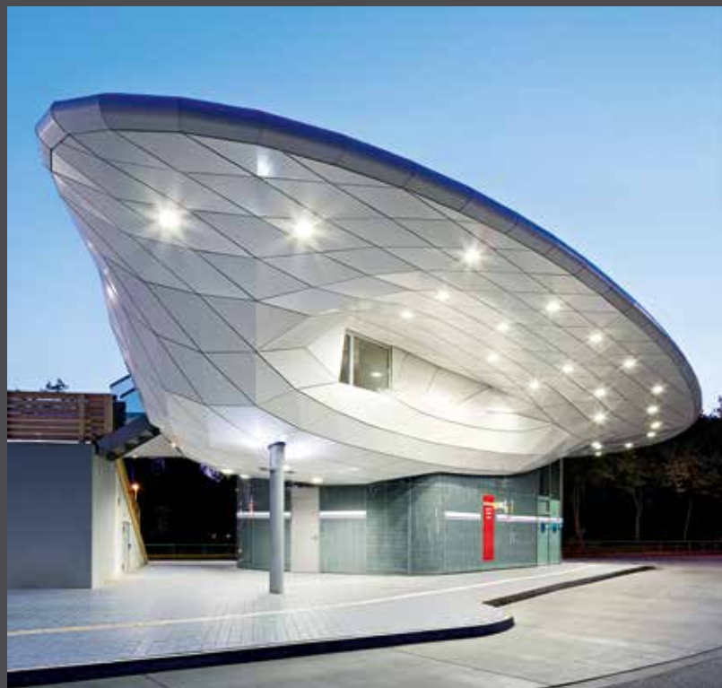
Poppenbüttel Bus Station's floating wing-shaped roof, made of ALUCOBOND® PLUS pure white. | Picture: archimages
