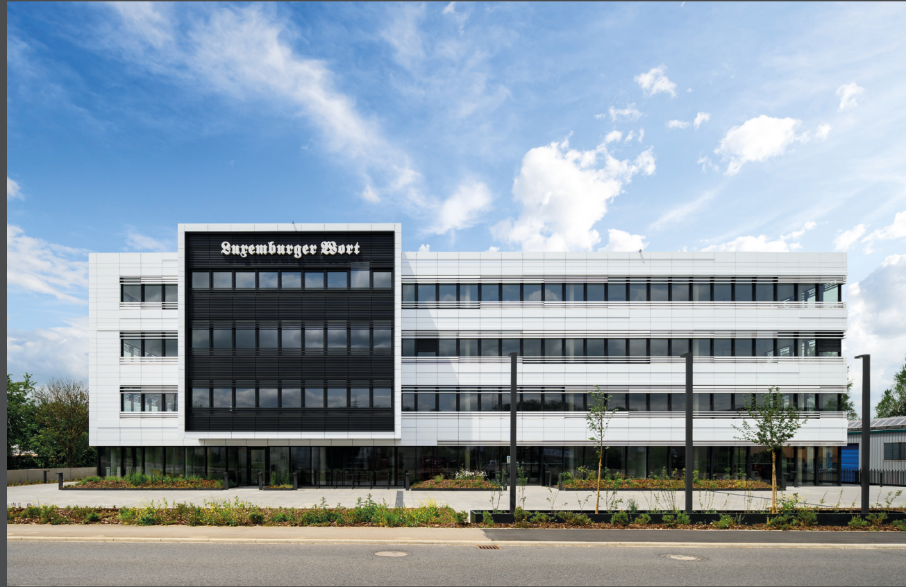
Luxemburger Wort, Luxembourg | Architect: M3 Architectes | Material: ALUCOBOND® PLUS White 16 | © Julien Swol
