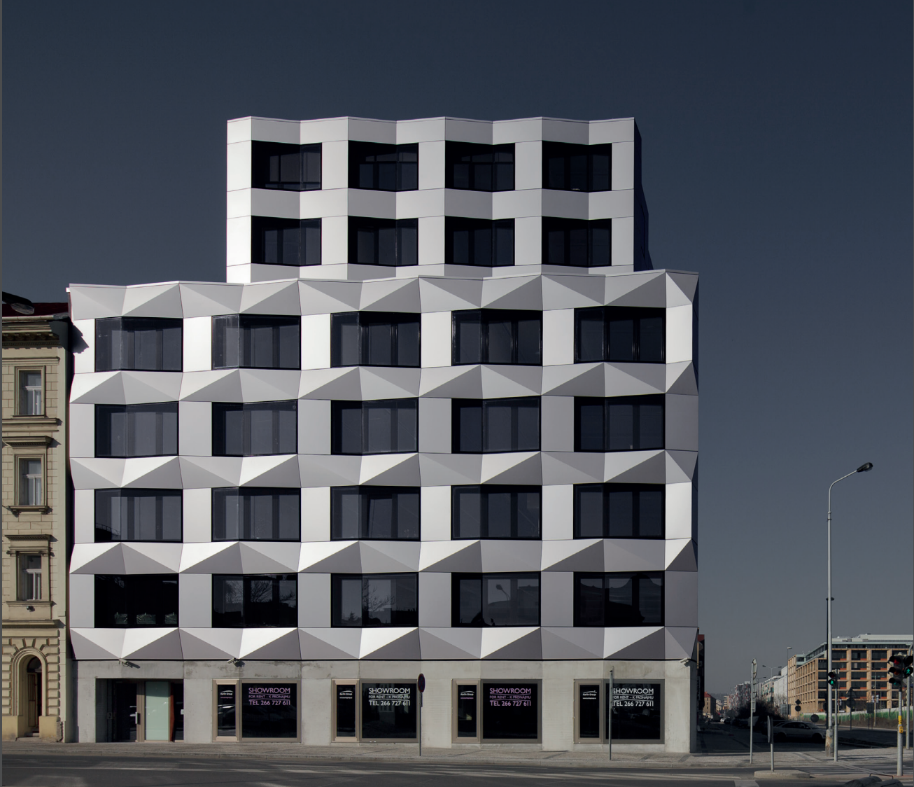
Keystone Office Prague, Czech Republic | Architect: EM2N, Mathias Müller, Daniel Niggli, Architekten AG, Zurich | Material: ALUCOBOND® A2 anodized look C0/EV1 | © Simon Menges
